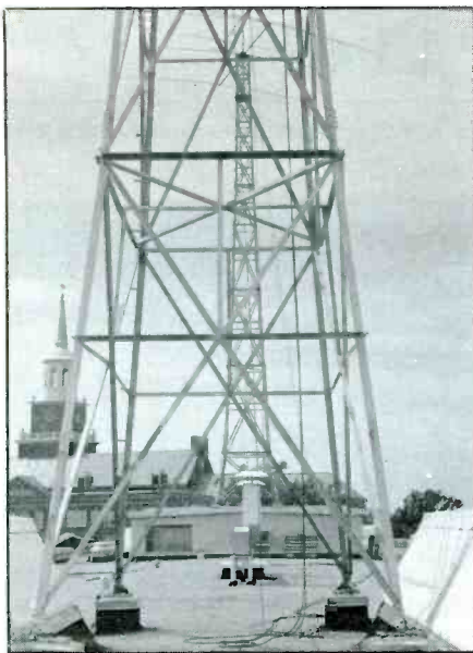
The W8YX towers as they look today. They're the same ones in the 1930 photo. (Courtesy Mark Milliron.)
